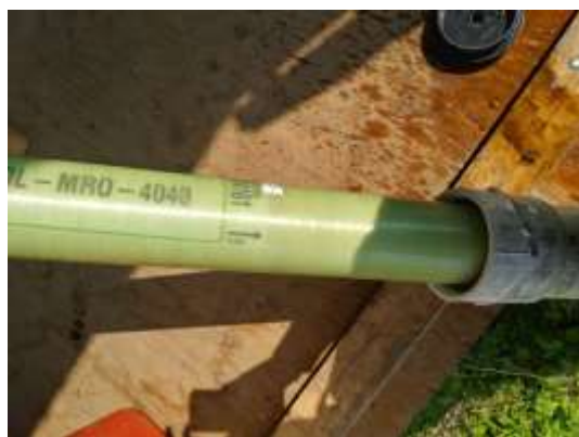
Figure 9.3: Arrow indicating flow on membrane housing
