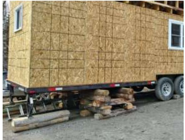
Figure 1: Trailer must be safely levelled
