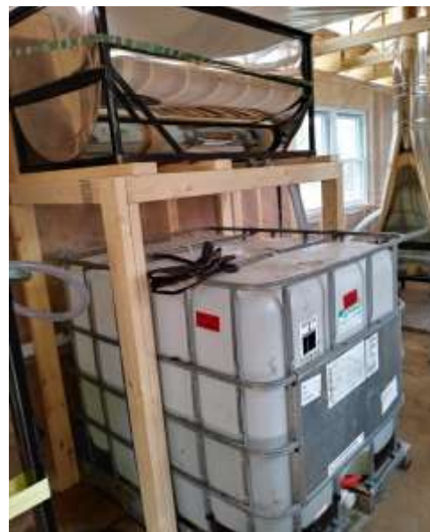
Figure 10.1: Concentrate goes on top, permeate goes in tank below
