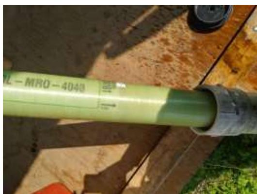
Figure 9.3: Arrow indicating flow on membrane housing
