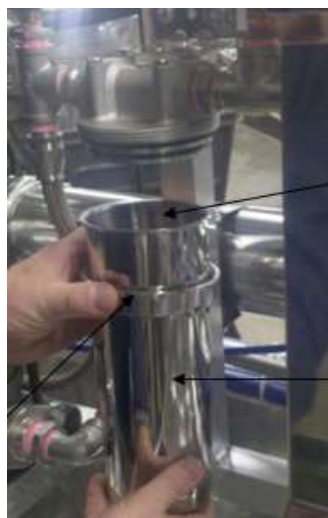
Figure 11: installing a pre-filter
